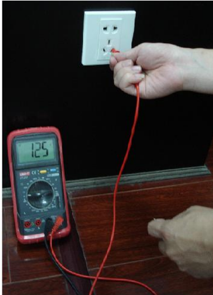
Appendix Figure 7-6 Check live cable connection
